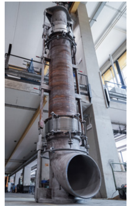
8 metres long and 3.2 tons in weight – a lateral expansion joint in maintenance
